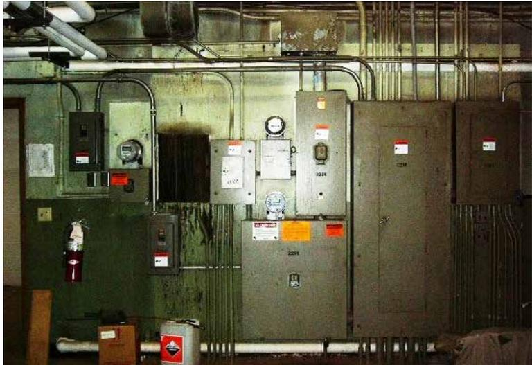
*Figure 3 – Electrical Service located in a Boiler Room showing equipment added for various building expansions.*
