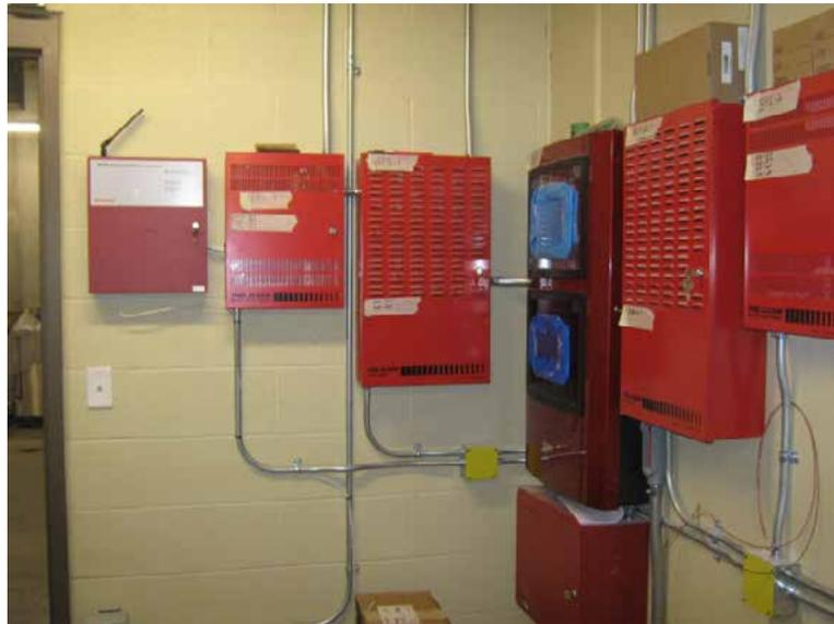
Figure 8 – Fire Alarm System
