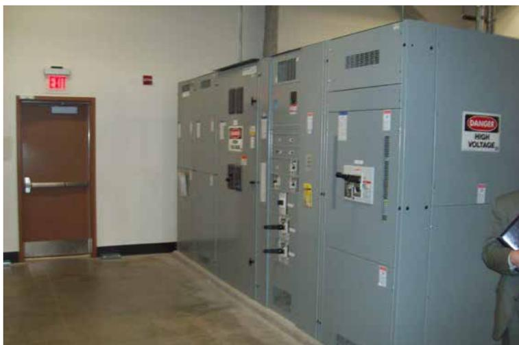
Figure 5 – Main switchboard with spare breakers and spaces and located in a dedicated electrical room.
