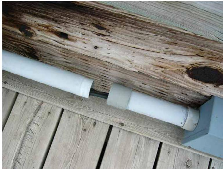
Figure 2 - Exterior PVC conduit pulled apart due to expansion and contraction due to heat.
