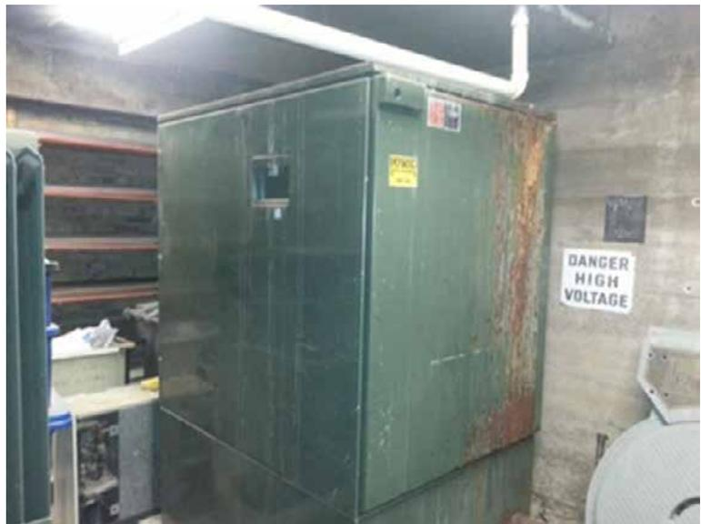
*Figure 4 – Medium volt switch in crawl space with significant corrosion after being exposed to a water leak for about 30 years.*
